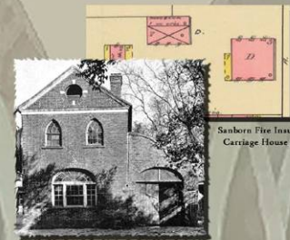
HABS Photo - Carriage House @ 18 Bull Street
