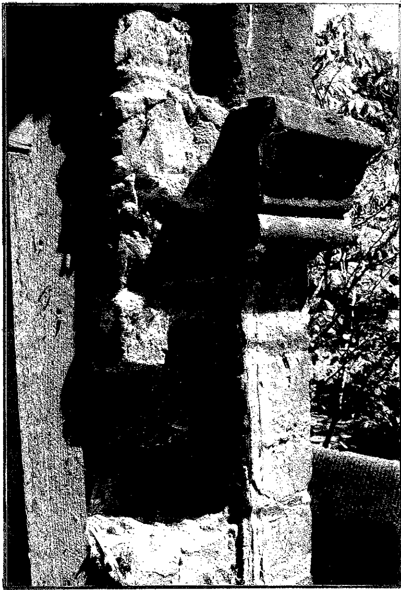
CONCRETE CORBELING MOISTURE PROBLEM
