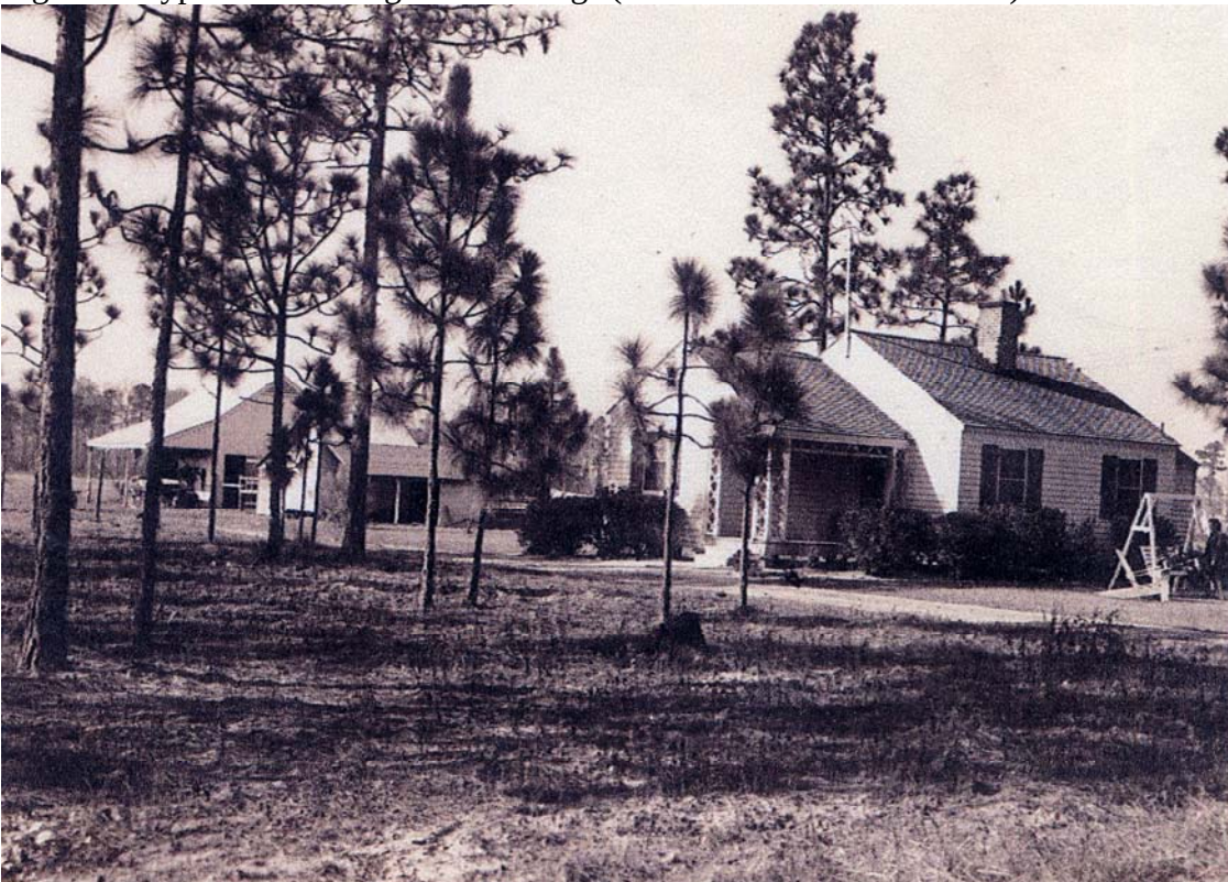
Figure 4: Typical assemblage of Buildings (Source: Penderlea Museum)
