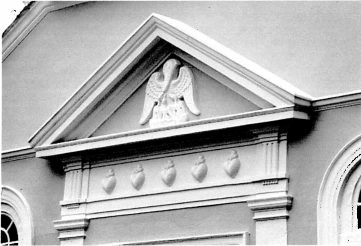
Fig. 5 – Pediment detail of St. James Church, St. James Parish, Berkeley County
