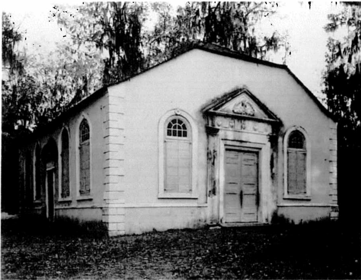
Fig. 4 – St. James Church, St. James Parish, Berkeley County
